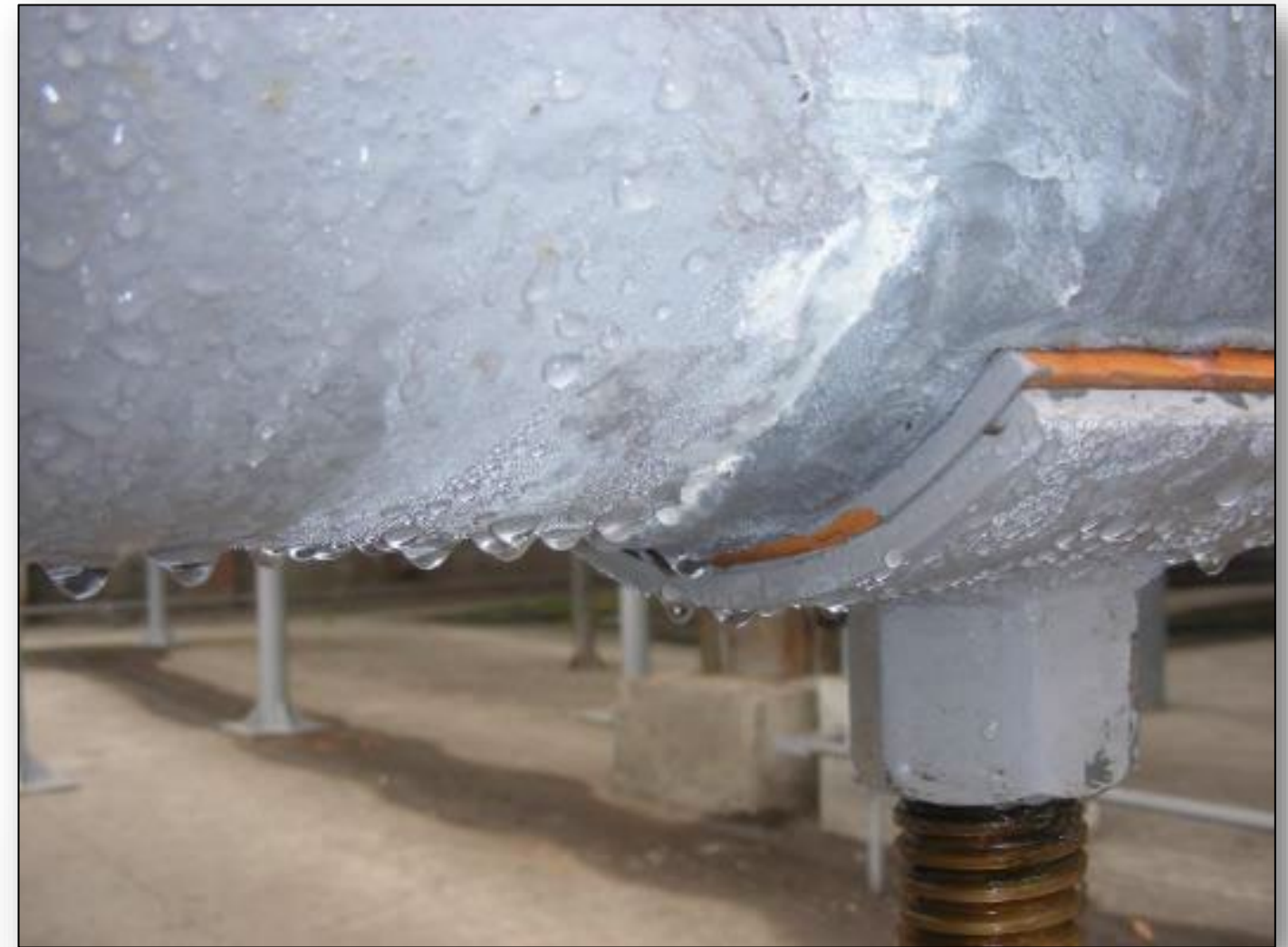
Condensing Pipelines
